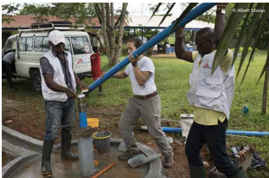
MSF water and sanitation experts install a hand-operated water pump at Abgokim clinic in Cross River state, Nigeria, November 2018.
